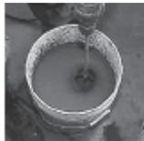
storm drain inlets during the saw-cutting operation and contain the slurry. Collect the slurry residue from the pavement or gutter and remove from the site.
